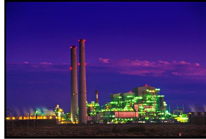
APS Cholla Power Plant,
