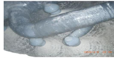
Fig. 8 Overlapping High Density Spray Patterns
