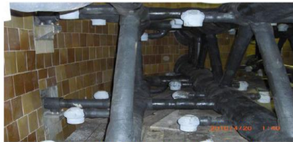
Fig. 7 Typical Spray Headers
